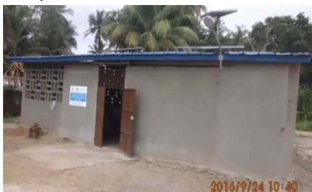
Figure 10. Secured shed housing the FTT processing facility at Braffedon
